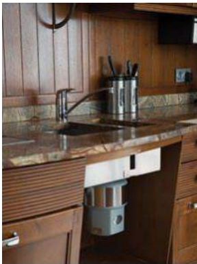
Disposer under the sink
